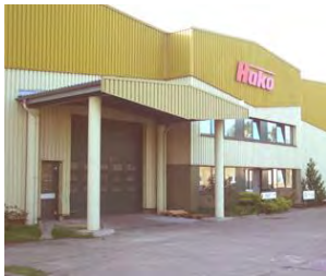
Hako manufacturing branch in Glindow /Potsdam, Germany
