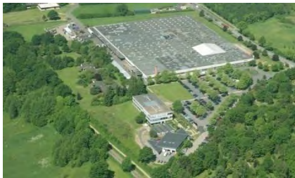
Hako-Werke GmbH main factory site and head office Bad Oldesloe, Germany
